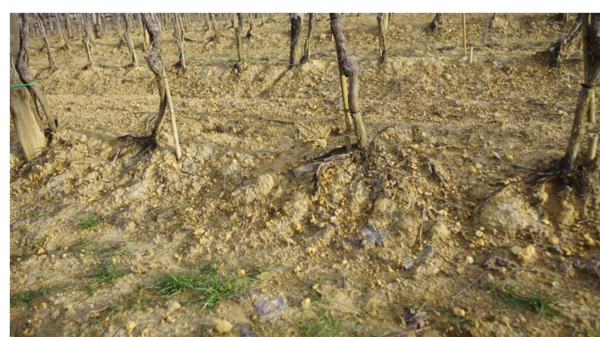
Fig. 1. Soil erosion/exposed roots.
